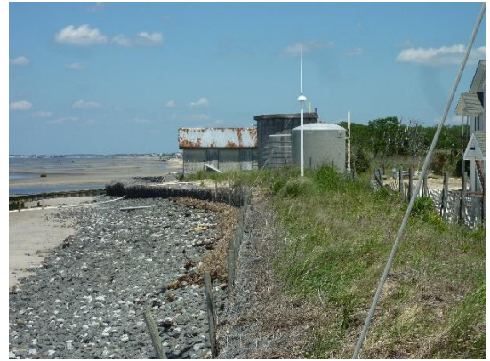
Shack which was the original research facility
